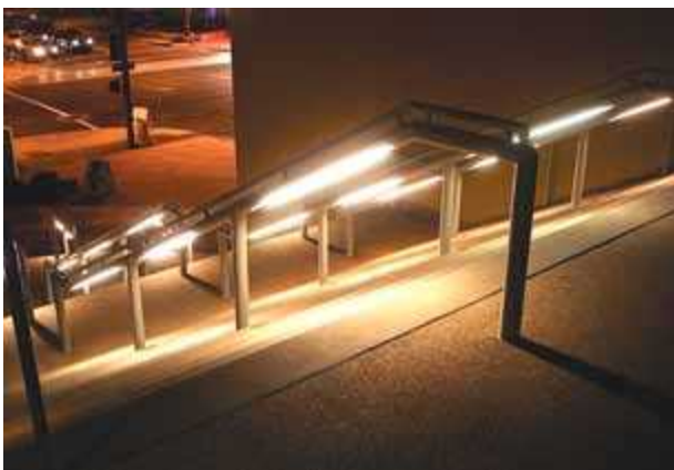
Exterior stair illumination via lights in stair handrail. (Courtesy of Jake Pauls)
