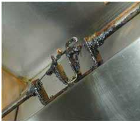
Fusible link requiring replacement.
