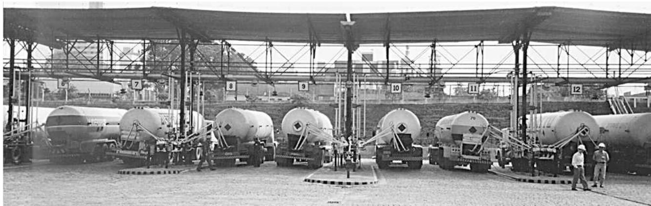
Transport trailers loading at a pipeline terminal.
