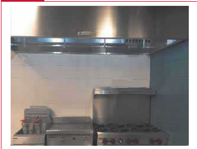
Hood suppression system. (Courtesy of Tyco Fire Protection Products)
