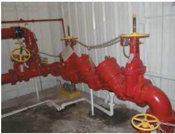
RPZ backflow prevention device. (Courtesy of Aon Fire Protection Engineering)
