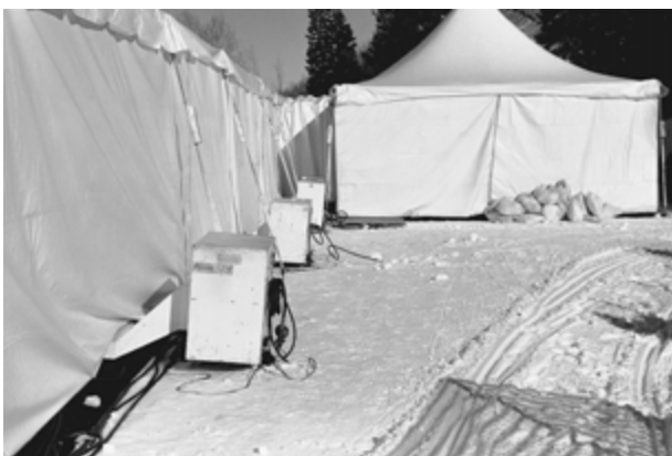
Portable heaters placed outside membrane structure.
