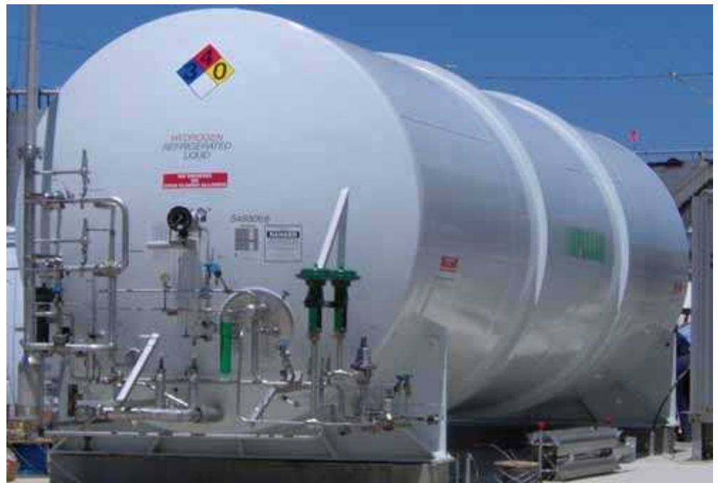
Signage on cryogenic fluid container.
