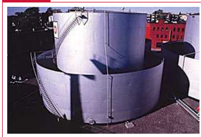
Diked tank to which 66.22.11.2.5(1) applies.
