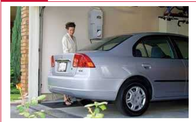
A residential CNG refueling system. (Courtesy of cleanenergyfuels.com)
