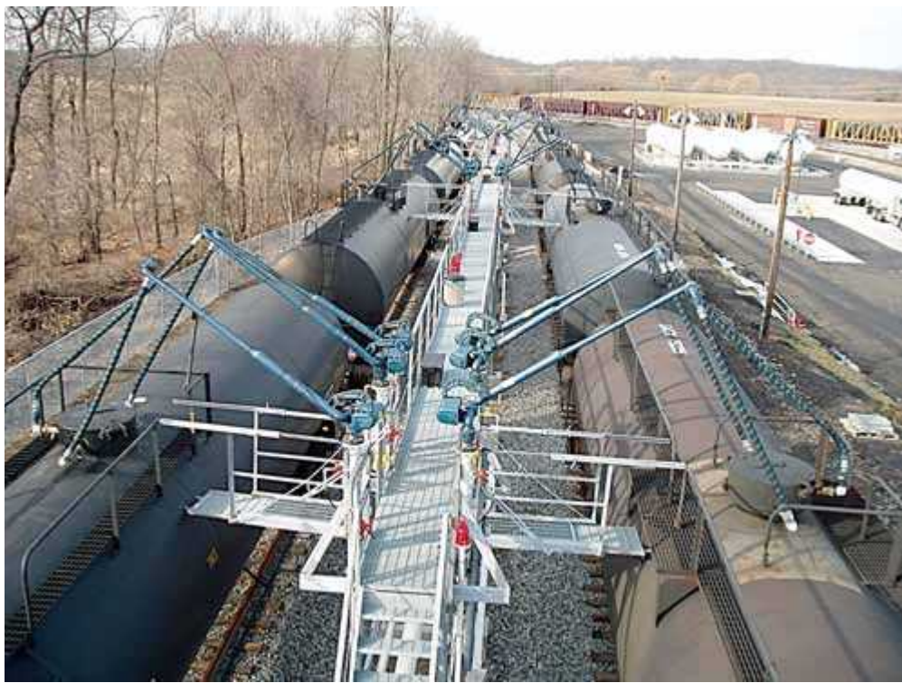
Tank car loading/unloading facility. Note the swing arms connected to the tank car dome. (Courtesy of Eastern Propane Corp.)
