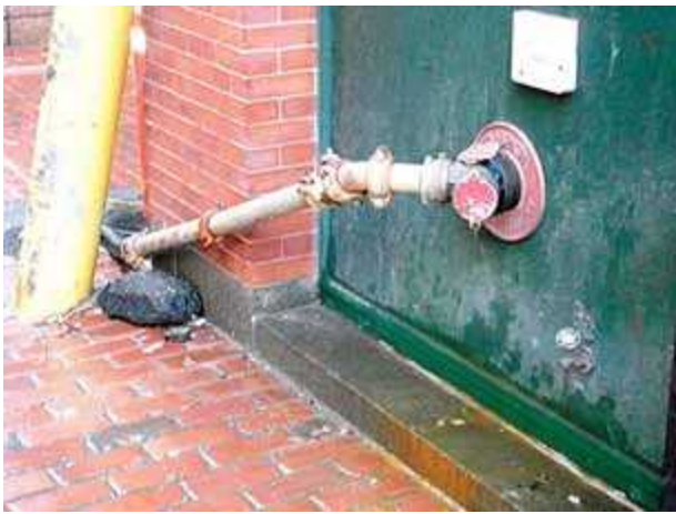
Temporary water supply connection to FDC.
