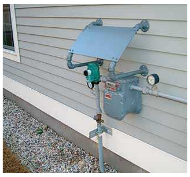
A method of meter protection in heavy snow areas. (Courtesy of Dead River Company)
