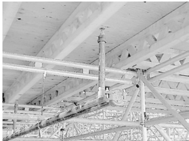
Sprinklers installed under a grandstand.
