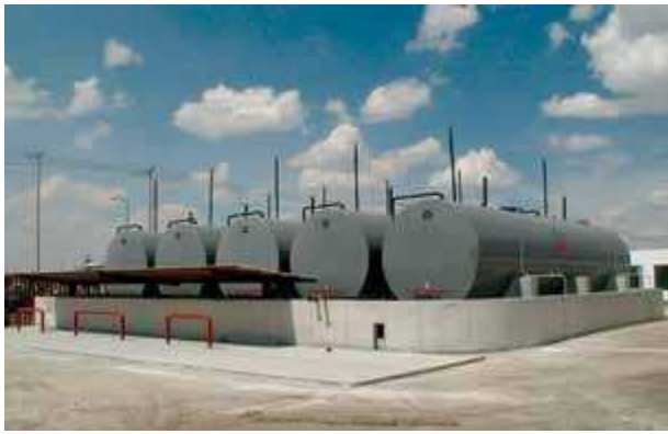
Horizontal aboveground atmospheric storage tanks.
