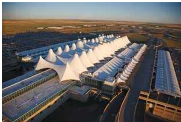
Membrane structure. (Courtesy of Denver International Airport)
