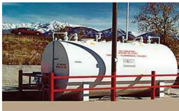
Collision protection for an aboveground storage tank. (Courtesy of Steel Tank Institute)
