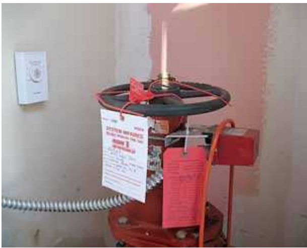
Example of an impaired system tag. (Courtesy of Byron Blake and SimplexGrinnell)
