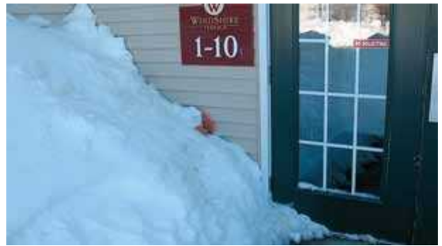
FDC obstructed by snow. (Courtesy of Byron Blake and SimplexGrinnell)
