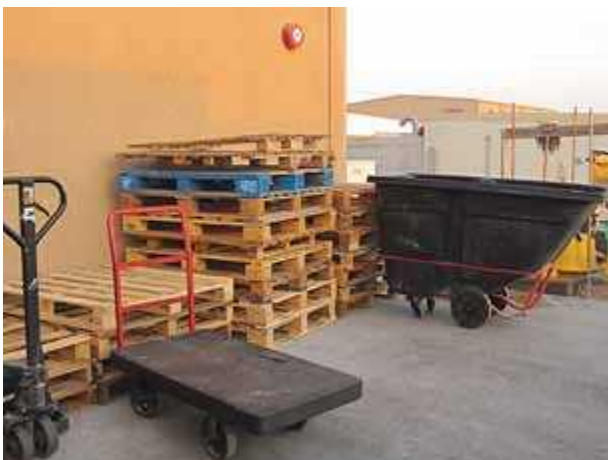
FDC obstructed and inaccessible due to exterior storage. (Courtesy of Byron Blake and SimplexGrinnell)
