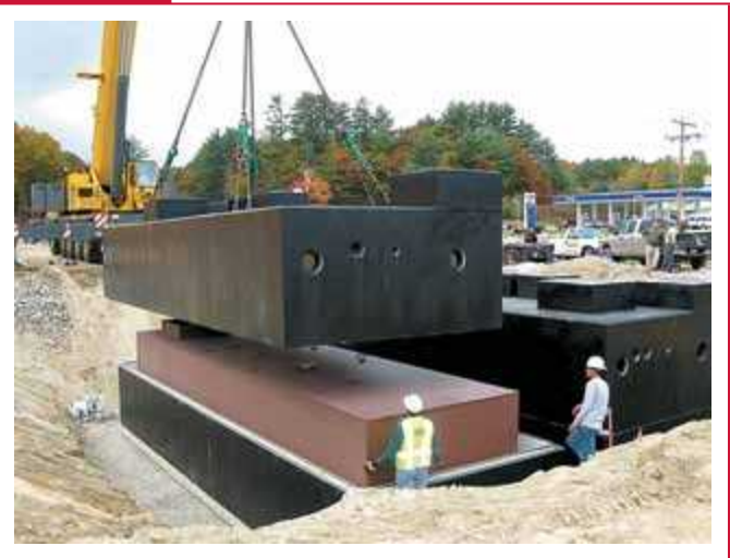
Vault and its storage tank being installed at a service station site. (Courtesy of Core Engineered Solutions, Inc.)
