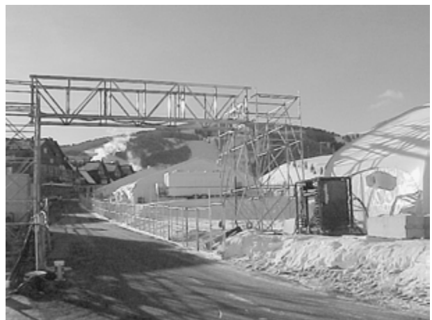
Elevated electrical system.
