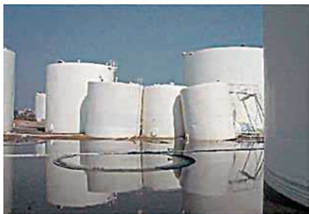
Storage tanks dislodged from their foundations due to Hurricane Katrina floodwaters.
