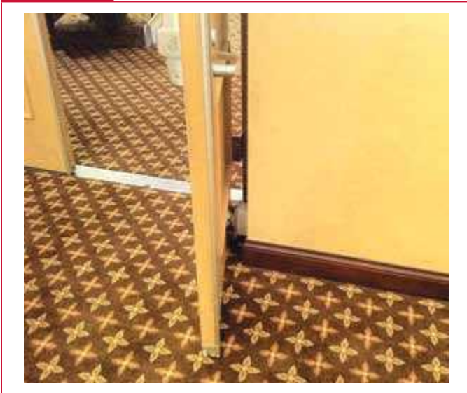
Automatic-closing door in open position.
