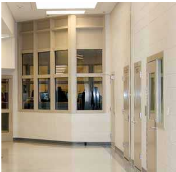
Glass-enclosed control rooms.
