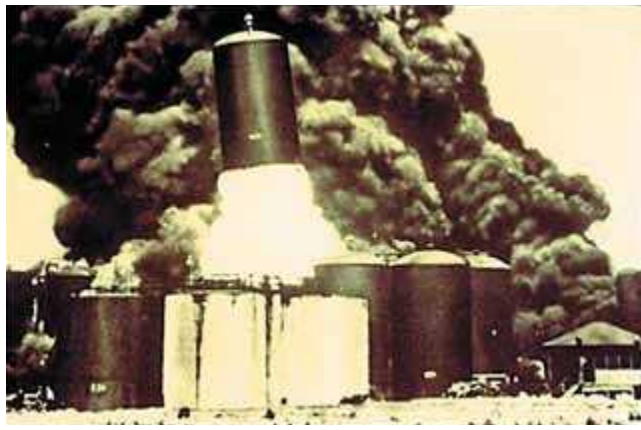
Catastrophic failure and rocketing of a tank due to inadequate emergency relief venting.
