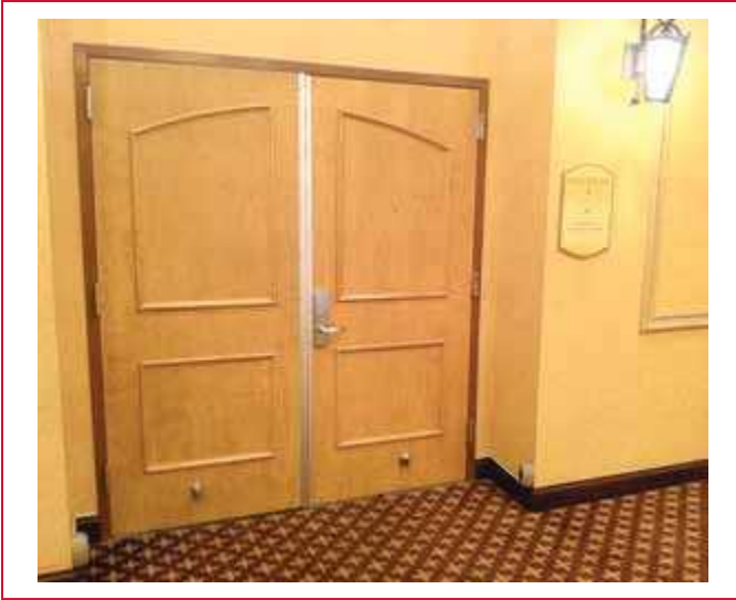
Automatic-closing door in closed position.
