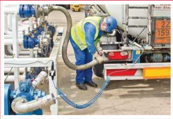
Bonding cable attached to a tank vehicle prior to loading cargo. (Courtesy of Newson Gale Inc.)
