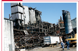
(Courtesy of the U.S. Chemical Safety Board)
