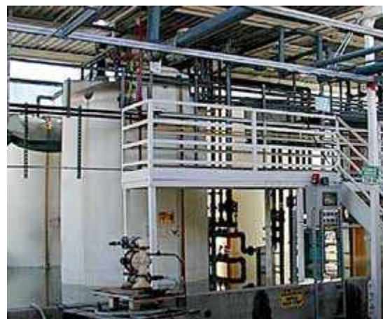
A typical chemical process plant.
