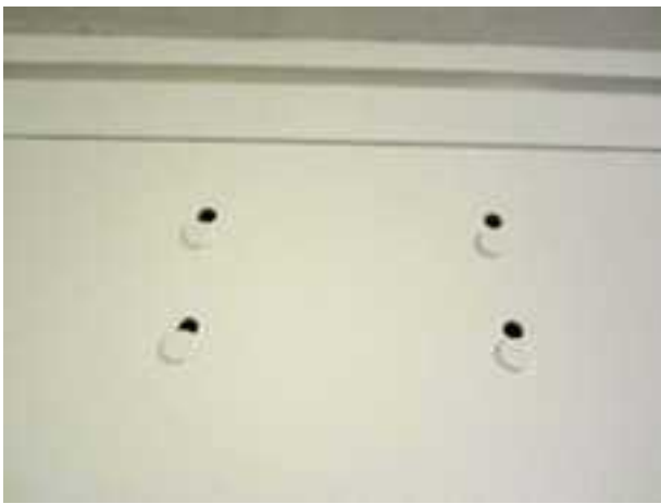
Fire door with an extra set of holes for installation of closing device. (Courtesy of Lori Greene)
