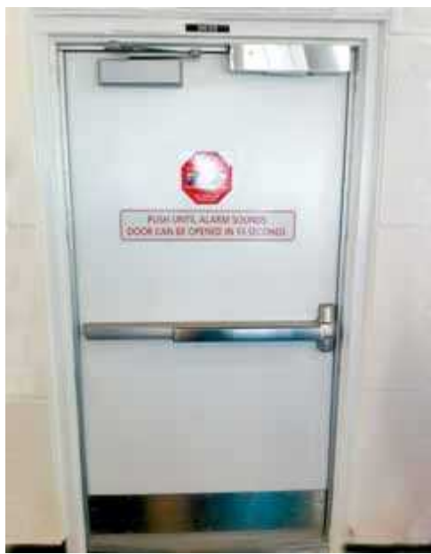
Delayed-egress electrical locking system hardware.
