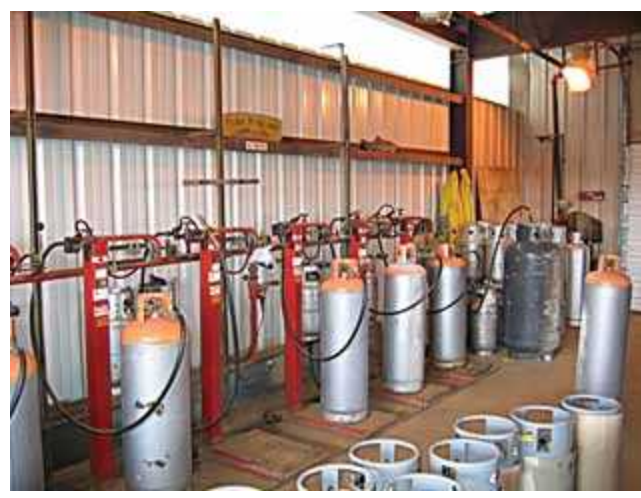
Cylinder filling room with automatic cylinder filling scales. (Courtesy of Propane Education and Research Council)
