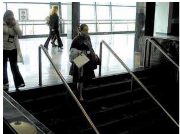
Poorly lit interior stair near brightly lit window space. (Courtesy of Jake Pauls)
