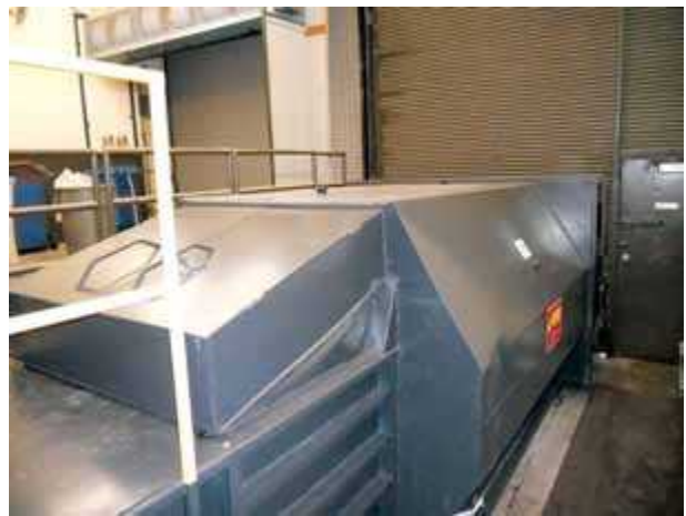
Large rubbish container in a protected room.
