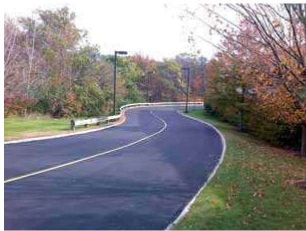
Fire department access road.
