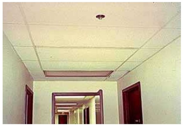
Retrofitted cross-corridor door that affects sprinkler spacing.
