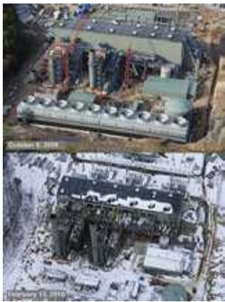
Kleen Energy plant before and after explosion. (Source: U.S. Chemical Safety Board)
