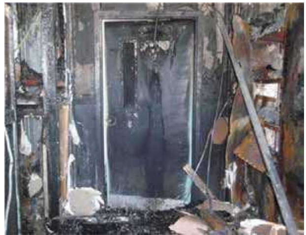
Fire door assembly from fire side.
