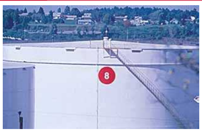
Closed-top floating roof tank.
