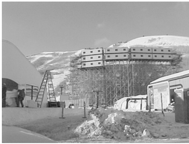
Temporary grandstand with enclosed spaces above.
