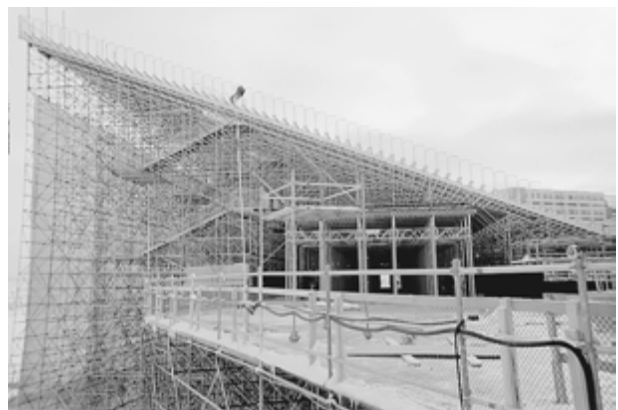
Large temporary grandstand.
