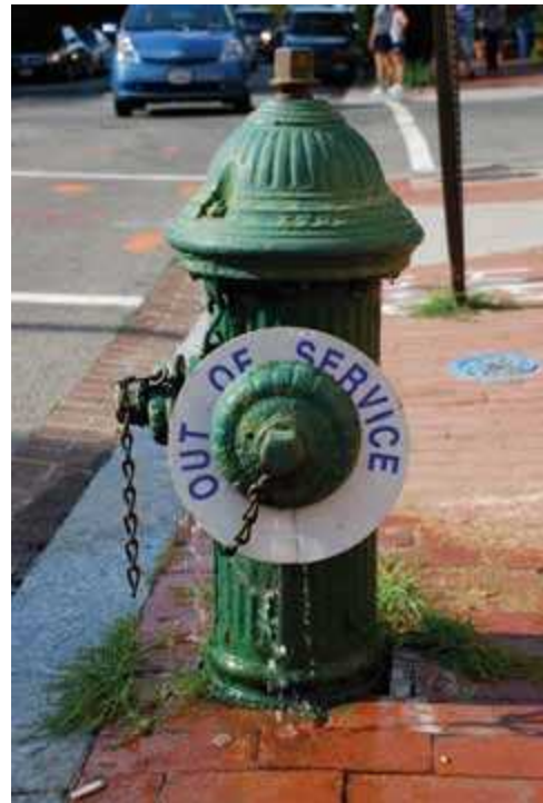
Fire hydrant with out of service indicator.
