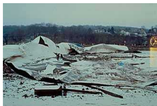
Destroyed oil storage tank, Floreffe, Pennsylvania, January 2, 1988.
