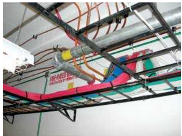
Cable penetrations through a fire barrier.
