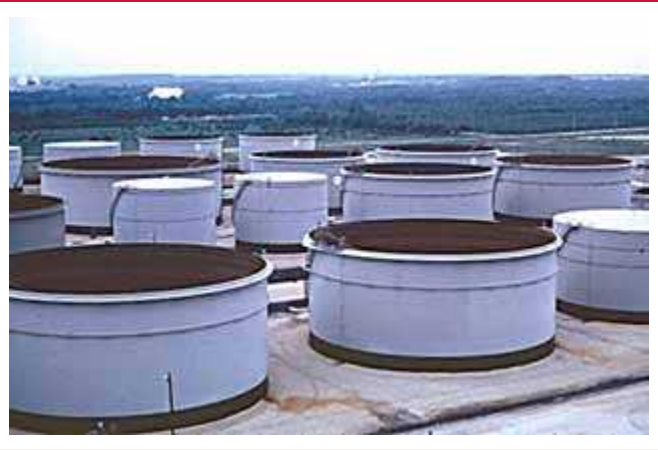
Open-top floating roof tanks.
